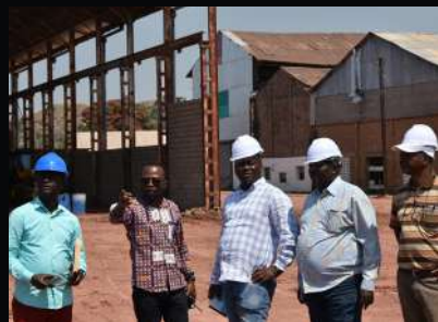
Control and monitoring of field work. Kalemie, September 2018
